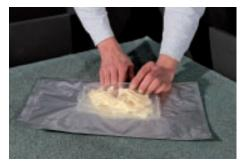
Carefully clean the dry surface to be patched, e.g. bitumen or PVC roof sheeting. Take out and put on the gloves.
