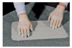
tear aid. Carefully pull out the KEMPEROL® 1K-SF Roofpatch. Apply to the area to be repaired, hold tight with one hand and pull the whole roof patch out of the aluminium bag. Smooth the roof patch with your hands to remove air bubbles and creases. That's it. The surface is rainproof in around 60 minutes.
